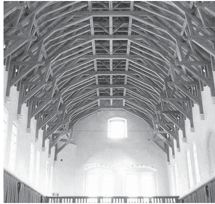
Figure i-3 Westminster Hall Hammer Beam Trusses
