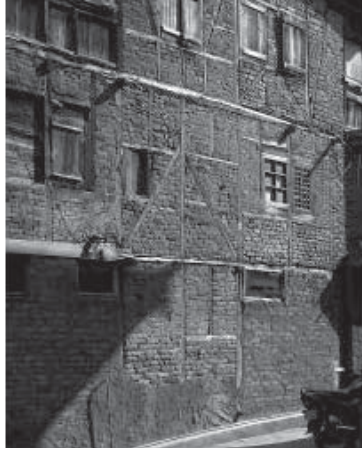
Figure i-2 Indian Post and Beam 'Dhajji-Dewari'
