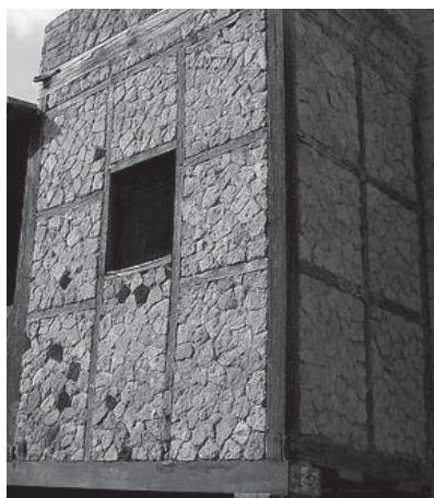
Figure i-1 Roman Post and Beam 'Opus Craticium'
