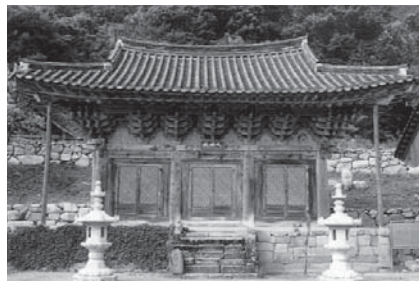
Figure i-3 Korean Post and Beam
